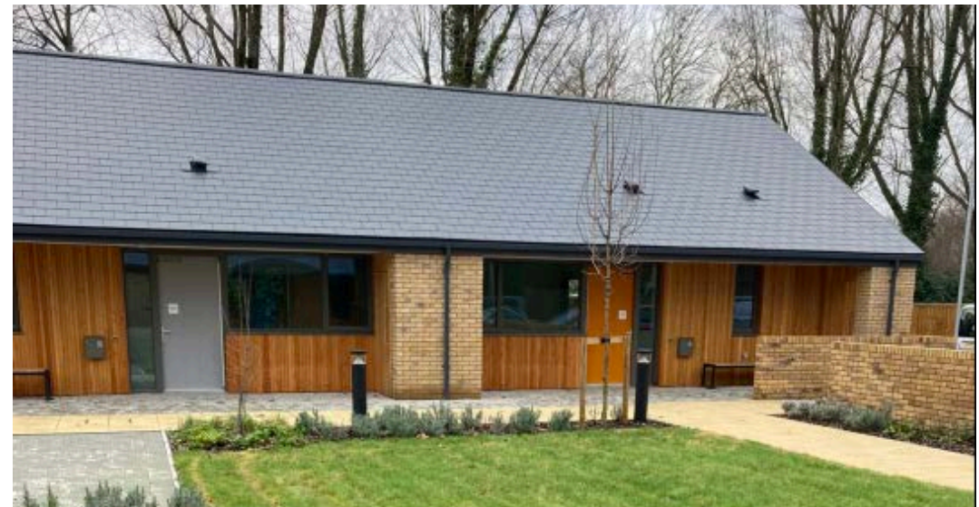
Newly developed homes at Sonnet Court, Hampshire
